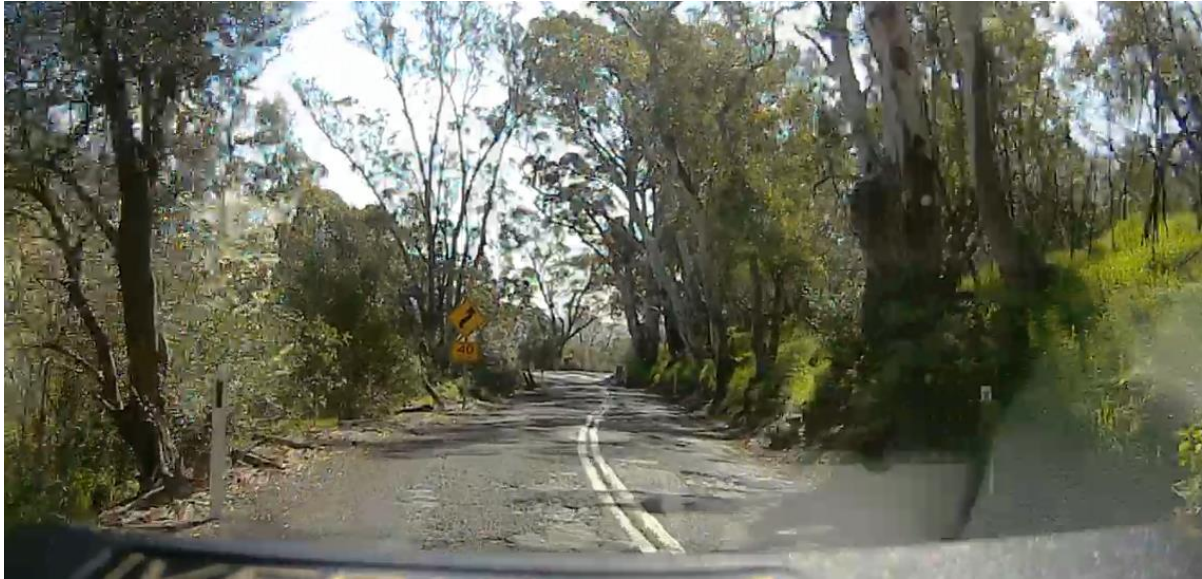
Figure 4: Deteriorating pavement and roadside hazards on Main Road
